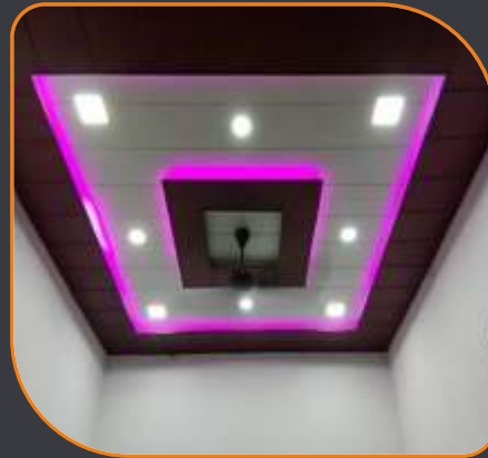
PVC False Ceiling
